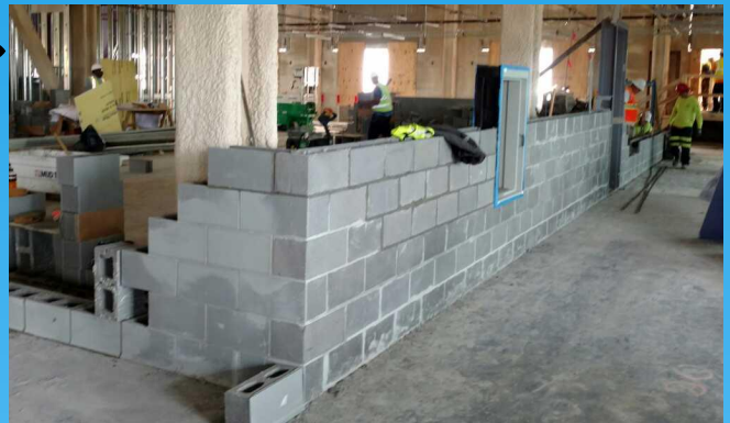
CMU Block Inside
