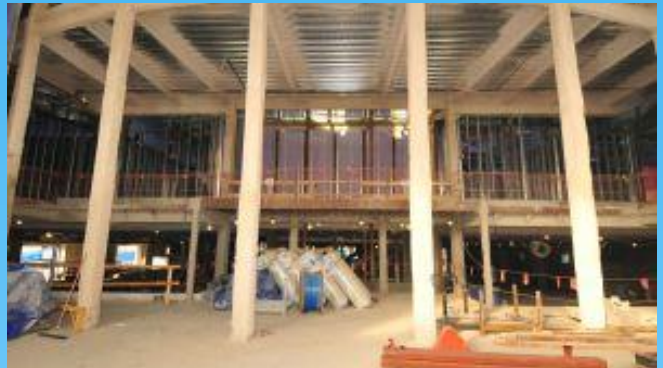
Main lobby level 1
