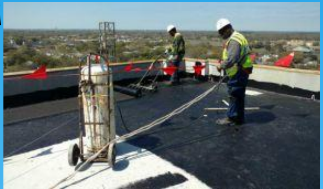
Temporary roofing installation
