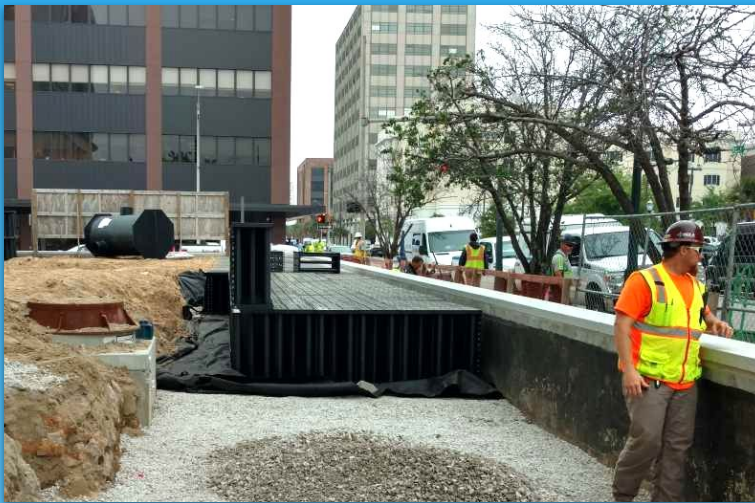
Stormwater tank module installation
