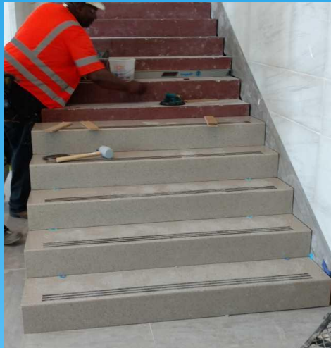
Lobby stair treads
