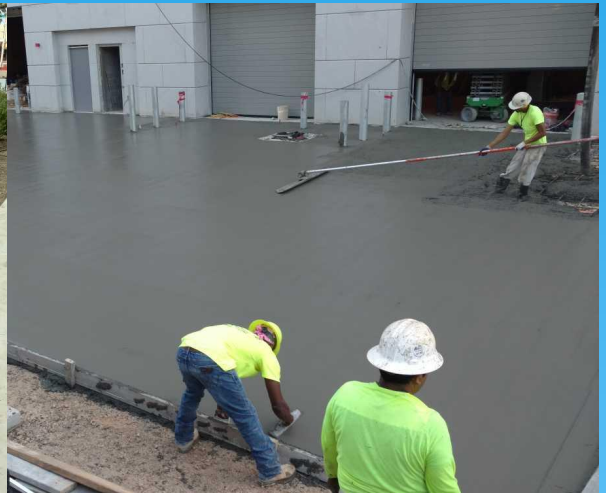
Floating the concrete service drive
