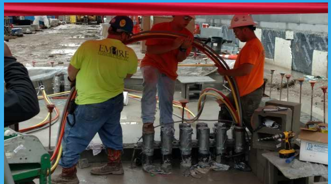
Electrical vault - pulling cables into building
