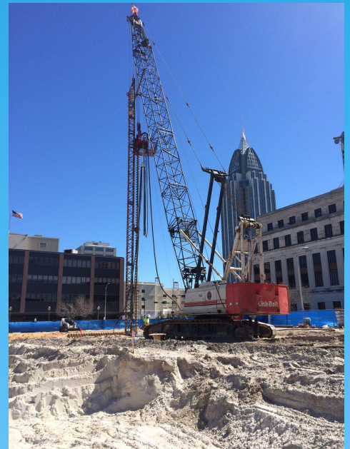
Crane used for setting piles
