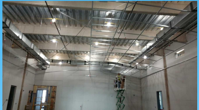
Vaulted ceiling in courtroom taking shape
