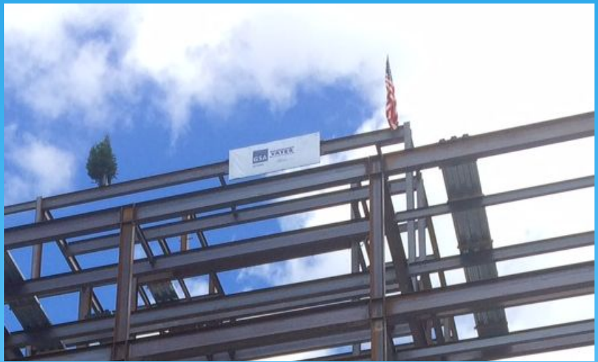
View of the last beam set on Sep. 14, 2016
