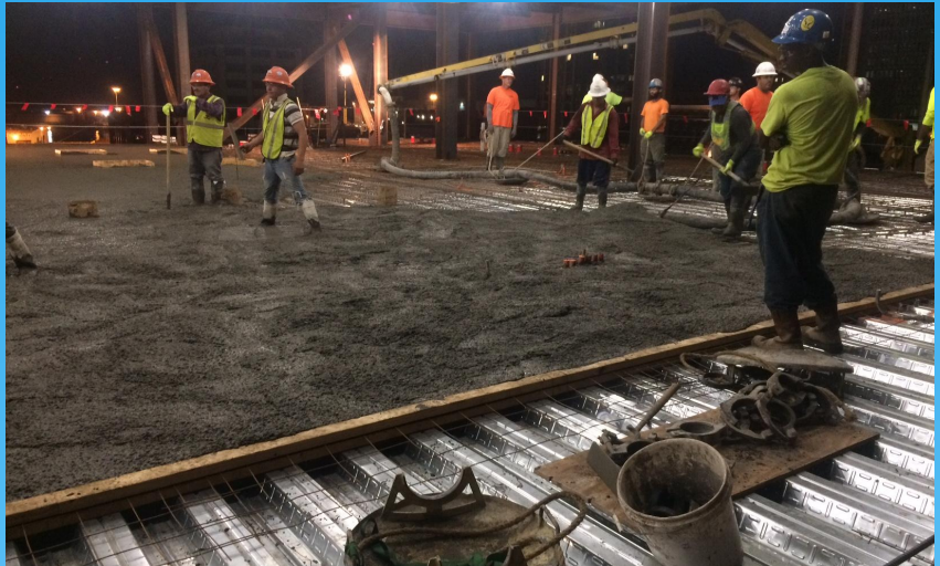
Placing concrete on metal deck 3rd floor
