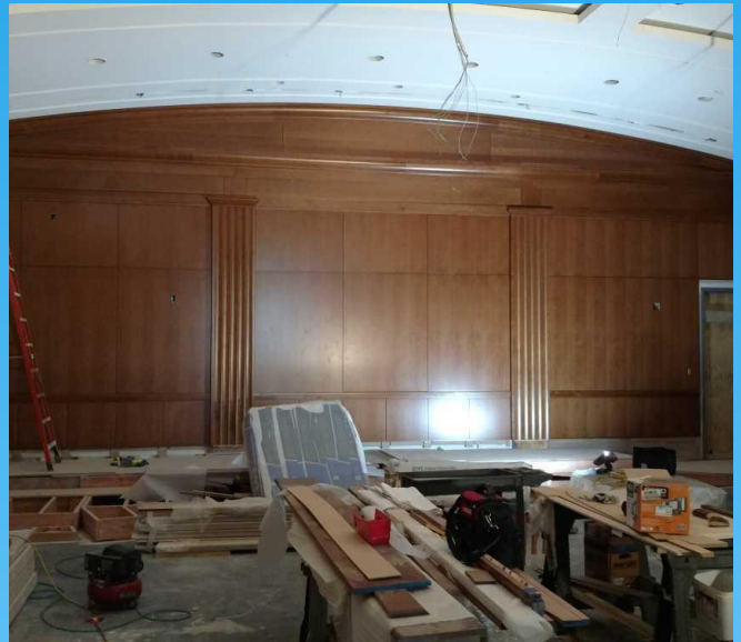
Courtroom millwork installation
