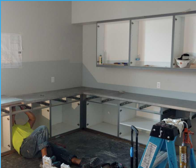
Casework installation
