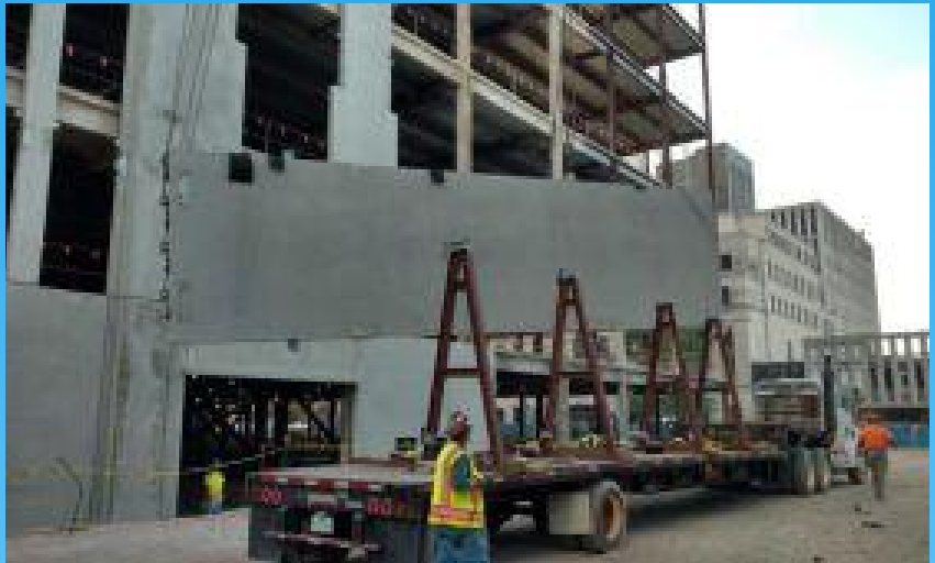
Lifting a precast panel off a flatbed truck
