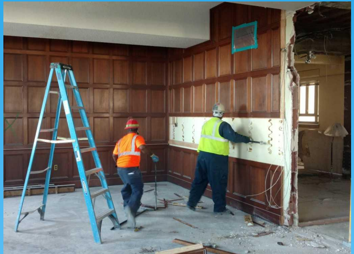
Deconstructing millwork wall panels
